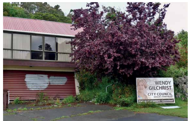
Fig. 2. A poster for Wendy Gilchrist, a candidate for the Hagley-Ferrymead Ward, displayed in front of a condemned house (Main Road, Mount Pleasant)
